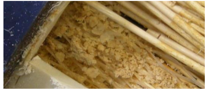
Carbonate scale deposits
