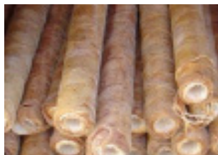
Fig 2: Iron fouled cartridge filters
